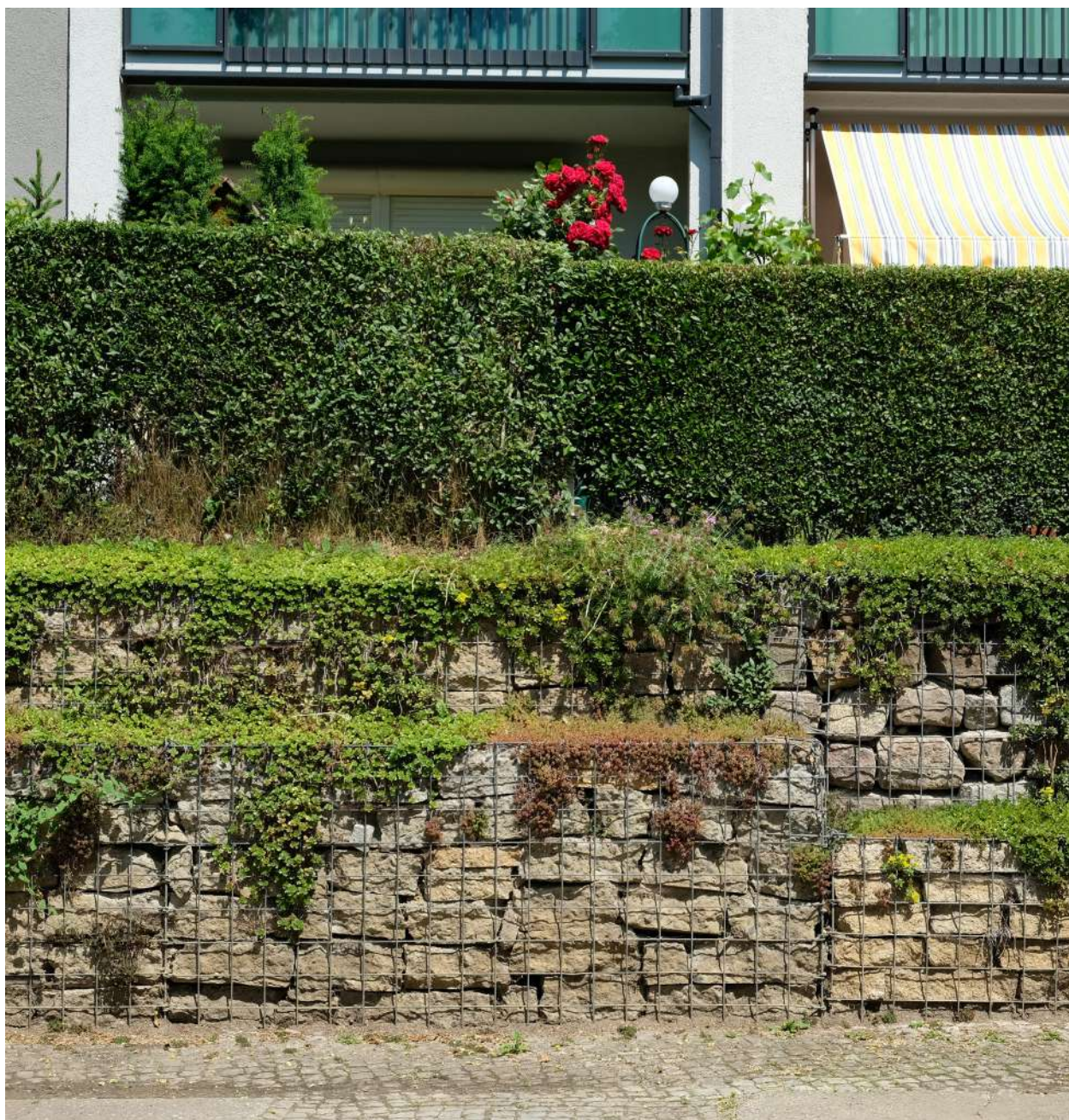
Fig 4.0 Planted stone gabions constructed using rubble from a demolished building in Berlin, Germany.
