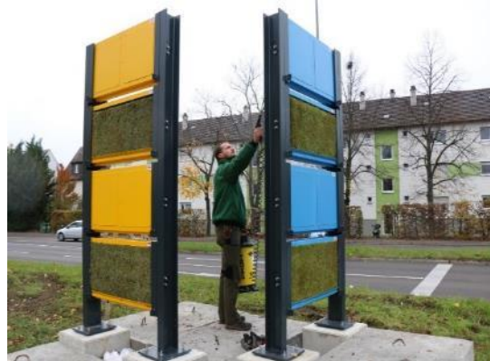
Fig. 40: MoosTex: Test site for pollution absorbing noise protection wall (source: Helix-Pflanzen)
