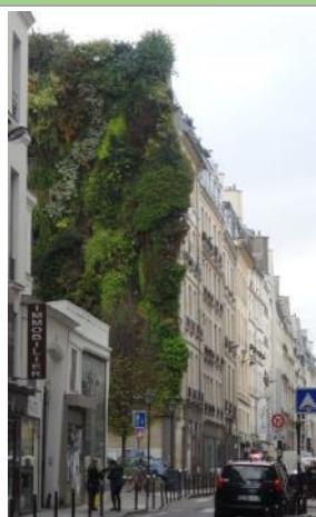
Fig. 32: Vertical Garden, façade-bound greening by Patrick Blanc, Paris (source: Eisenberg)
