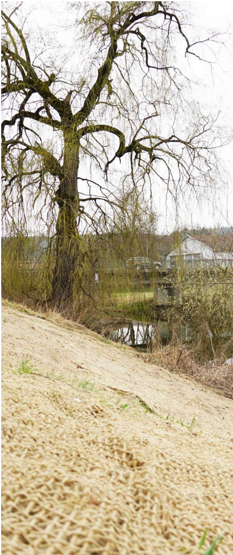
Fig 3.5 Planted embankment mat along the Danube river in Fridingen, Germany.
