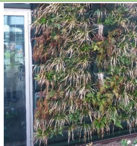
Fig. 34: Façade-bound greening, Amsterdam (source: City of Tampere)
