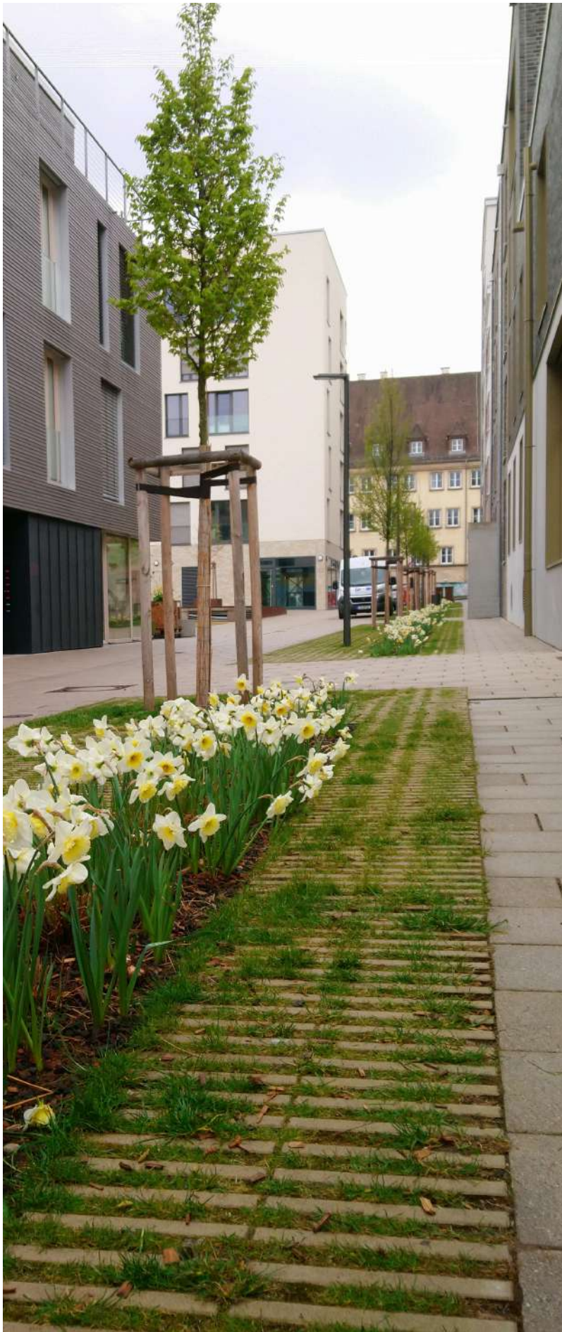
Fig 6.6 Permeable paving system in Stuttgart, Germany.
