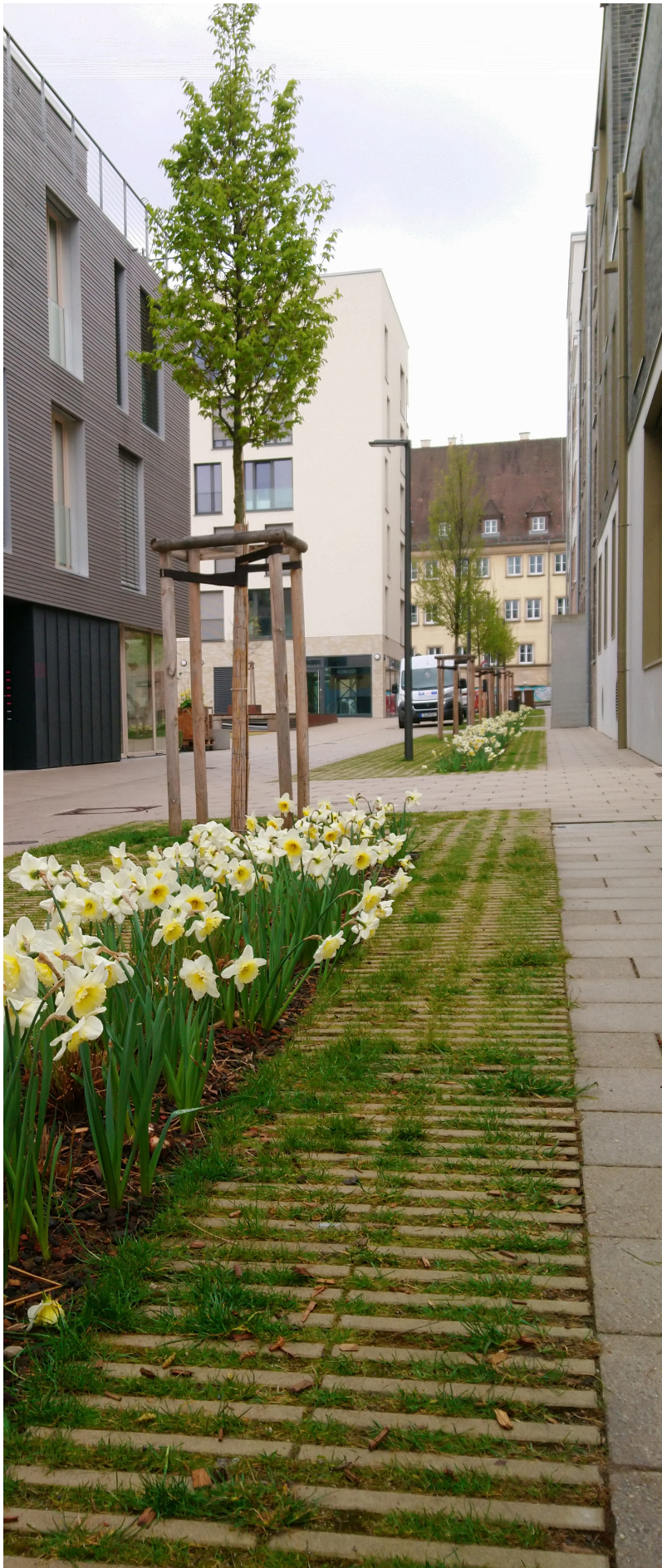
Fig 6.6 Permeable paving system in Stuttgart, Germany.
