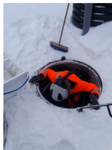
Taking calibration samples from automatic water measurement stations during winter.
