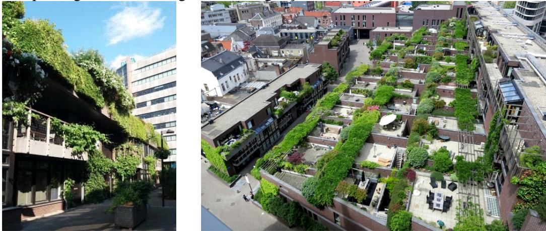
*Figure 2.6: Examples of green building façade and green roofs (Eindhoven, Medina)<sup>6</sup>*
