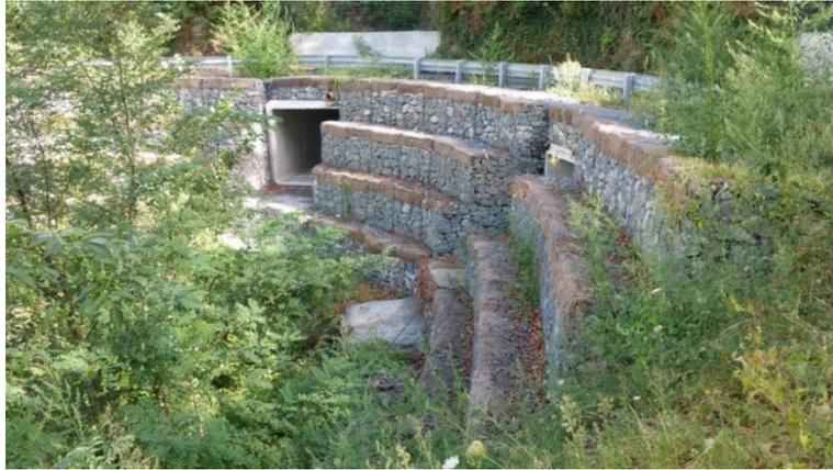
Figure 2.8: Example of Vegetated Gabion <sup>10</sup>
