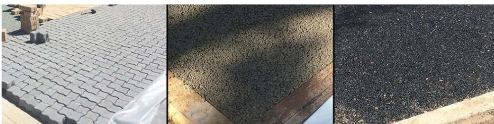
Figure 2.1: Pavement types - permeable pavers, permeable concrete and permeable asphalt
