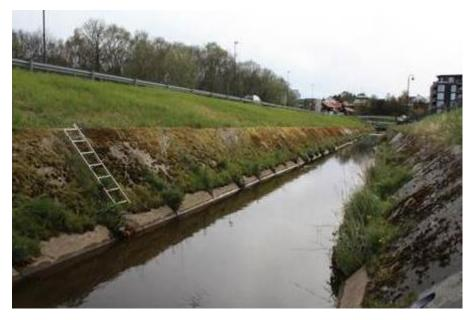
A typical cross section of the canal as it looks like at present. The idea of the Municipality of Stavanger is to remove the concrete and make a more riverlike system maintaining the current flow capacity.
