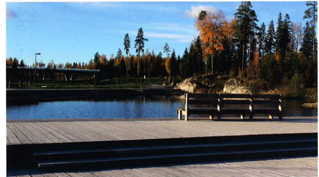
Figure 3. The heart of Vuores' nature-based stormwater management system is Central Park, where retention ponds (above), swales, and wetlands retain and purify waters before discharge to Lake Koipijärvi. Image © City of Tampere / Vuores
