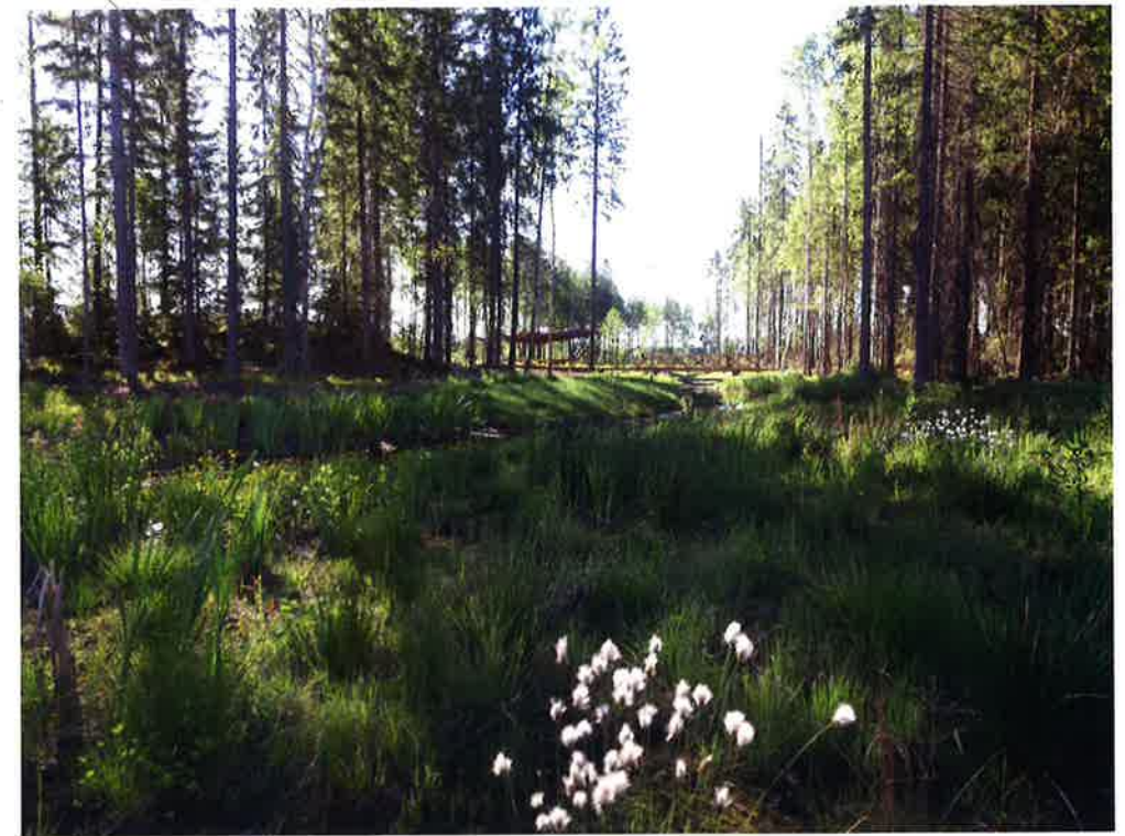
Figure 1. A constructed wetland in Vuores, Tampere, filters stormwater runoff to remove pollutants before discharge to the area's oligotrophic surface waters. Image © Maarit Särkilähti.
