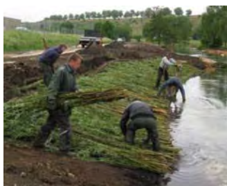
(b) Revetment under construction 28
