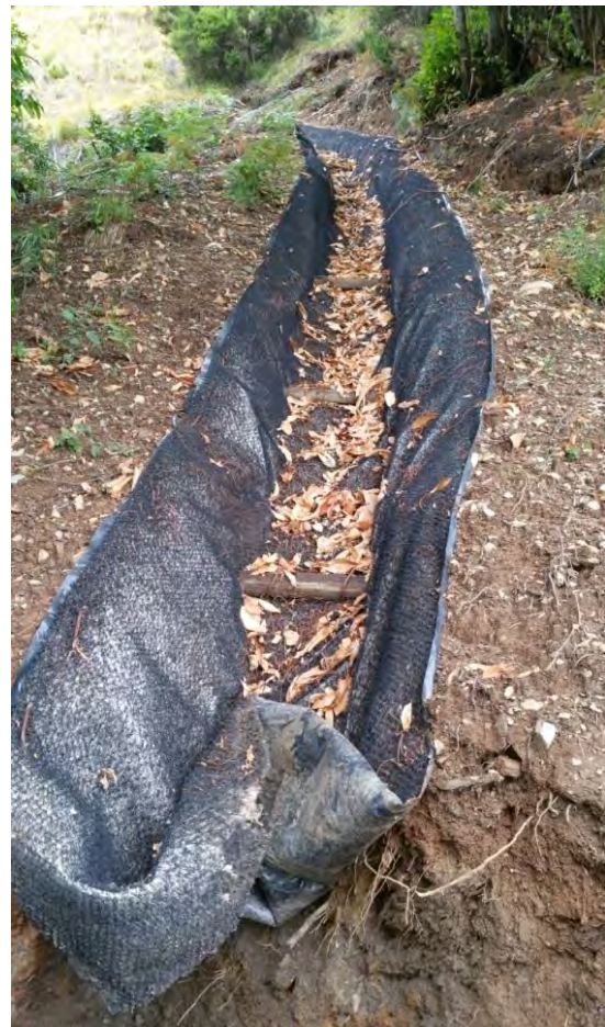
Figure 10.2: NBS solutions applied for meteoric water management [Provided and owned by the Municipality of Genoa]
