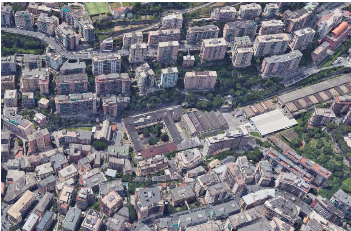
Figure 5.3: Aerial view of the Lagaccio neighbourhood [Source: https://www.google.com/maps/ ]
