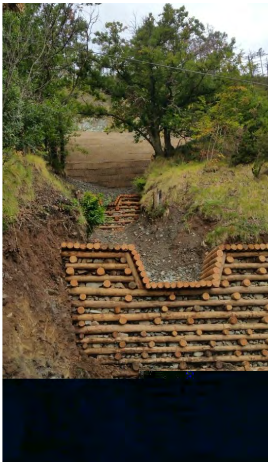
Figure 10.2: NBS solutions applied for meteoric water management [Provided and owned by the Municipality of Genoa]
