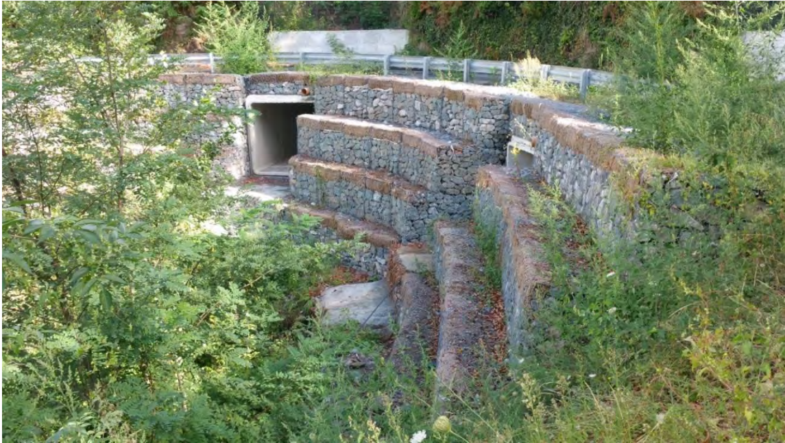
Figure 10.3: Example of vegetated gabion stones [Provided and owned by the Municipality of Genoa]
