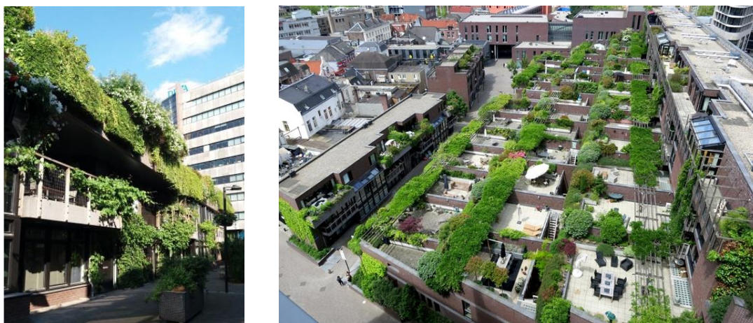
Figure 2.1: Examples of green building façade and green roofs (Eindhoven, Medina) 1
