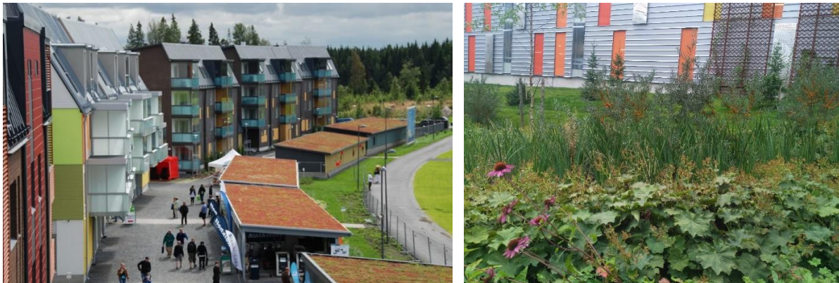
Figure 2.5: Examples of urban gardens with small-scale NBS in Tampere and Helsinki
