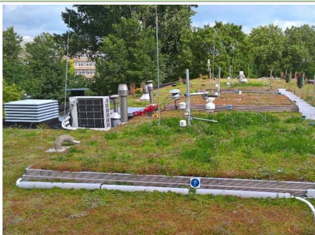
Fig. 42: "Polderdaken" (smart retention roof (source: Amsterdam Rainroof ; www.rainproof.nl)
