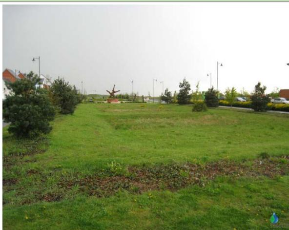
Fig. 49: Infiltration basin (source: [www.susdrain.org](http://www.susdrain.org))
