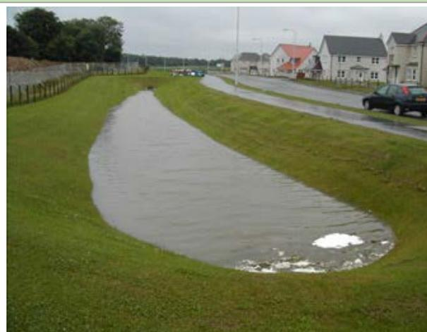
Fig. 53: Detention Pond (source: www.sudswales.com)
