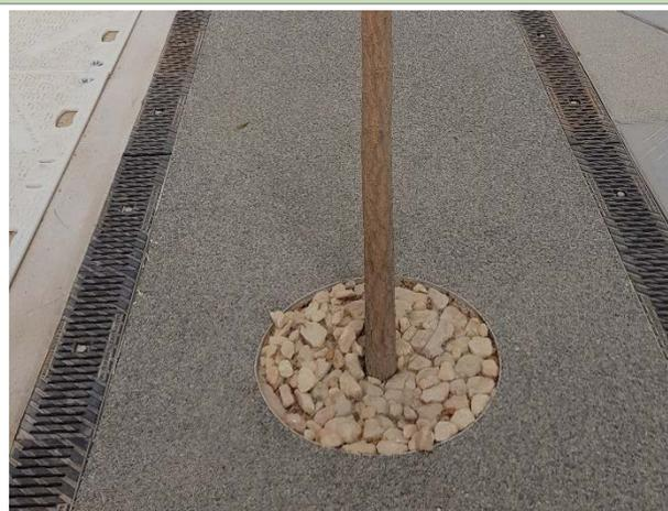
Fig. 66: Permeable stone carpet around a tree (source: LAND; <https://www.landsrl.com/>)
