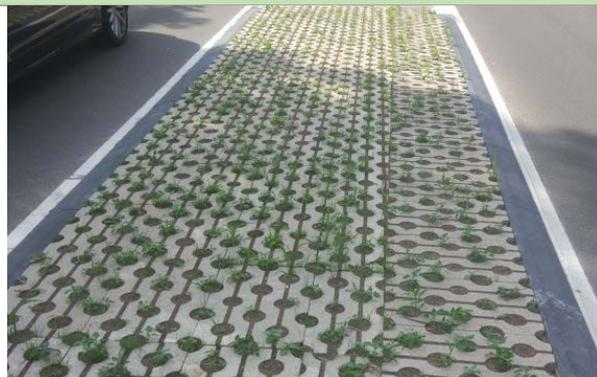
Fig. 61: Eindhoven, vegetated grid pave (source: Eisenberg)
