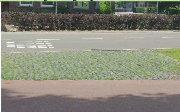
Fig. 60: Eindhoven, vegetated grid pave (source: Eisenberg)
