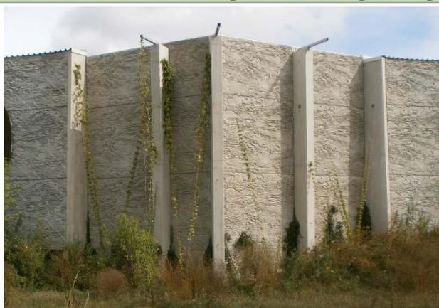
Fig. 23: Ground based greening on noise barrier (source: LAND; <https://www.landsrl.com/>)
