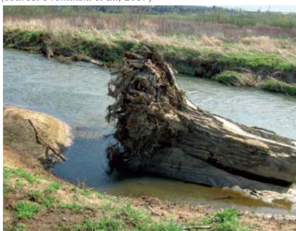
Fig. 92: Introducing disruptive elements in the Isar, Munich
