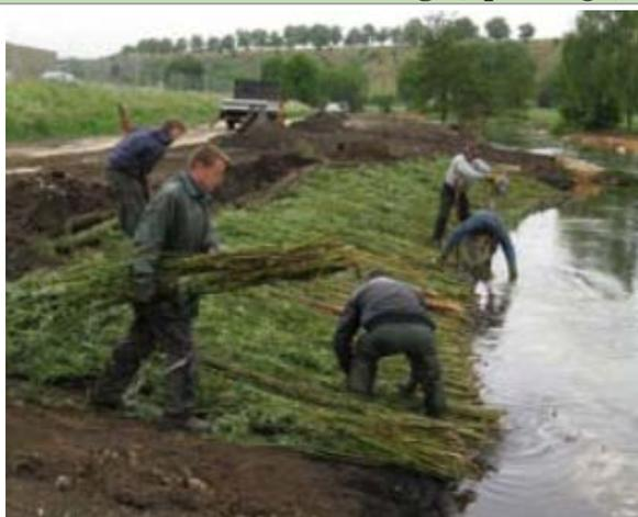
Fig. 100: Revetment under construction
