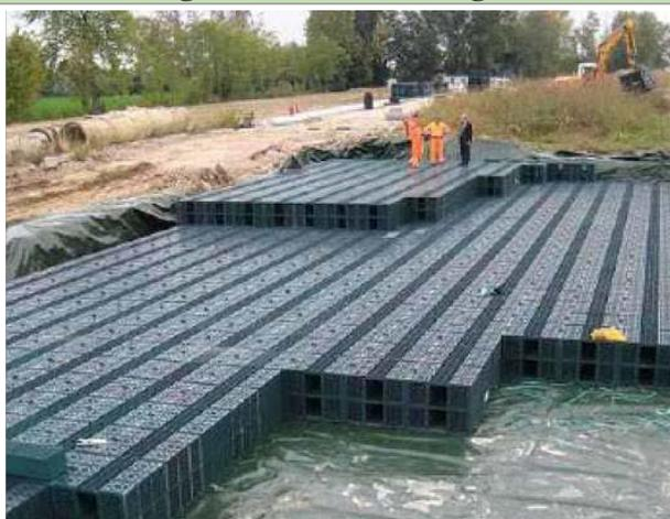
Fig. 67: Underground water storage (source: Commune di Genova)
