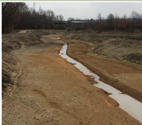
Fig. 78: Daylighting of a small stream in work (source: LAND; <https://www.landsrl.com/>)
