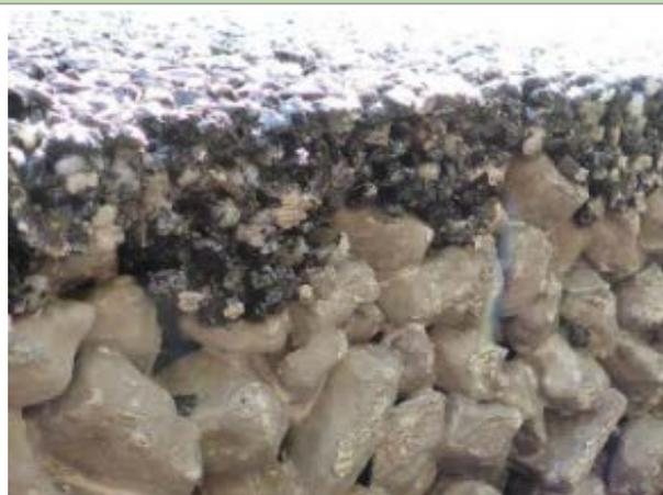
Fig. 63: Permeable concrete (source: New Dawn Permeable Paving P/L; [www.newdawnpermeablepaving.com.au](http://www.newdawnpermeablepaving.com.au))
