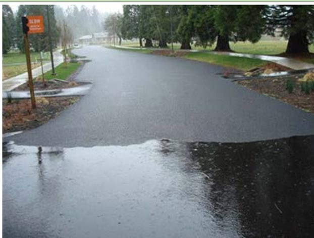
Fig. 64: Porous asphalt (source: New Dawn Permeable Paving P/L ; [www.newdawnpermeablepaving.com.au](http://www.newdawnpermeablepaving.com.au))
