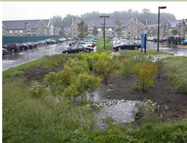
Fig. 50: Infiltration basin (source: SuDS Wales; [www.sudswales.com](http://www.sudswales.com))
