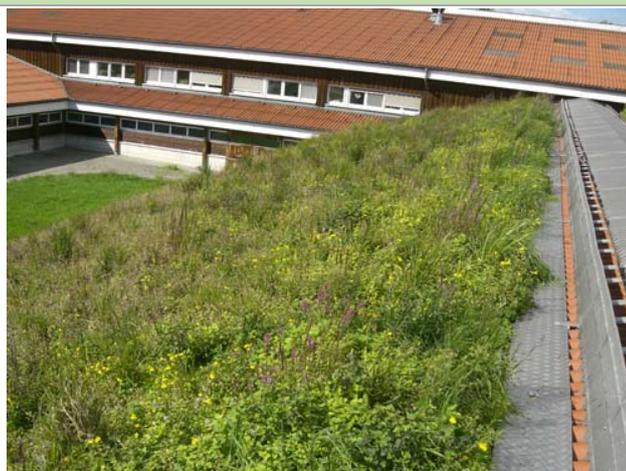
Fig. 45: Constructed wet roof (source: Rhizotech; www.rhizotech.com)
