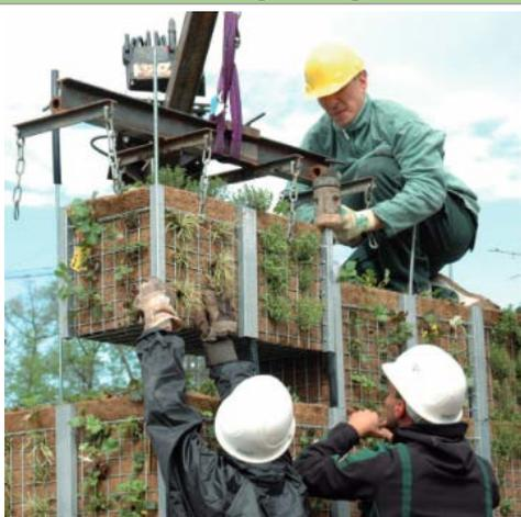
Fig. 25: Constructing a living wall, Ludwigsburg (source: (Helix Pflanzensysteme GmbH n.d.)
